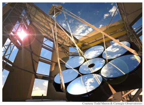
Plans call for the Giant Magellan Telescope, which is scheduled for completion in 2016, to be housed in a 213-foot-tall rotating enclosure. Seven 27.6-foot mirror segments would be combined to create a giant light-gathering instrument with up to 10 times the resolving power of the Hubble Space Telescope.
